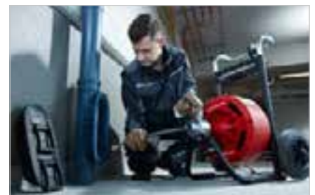
Cleaning of a down pipe with 16 mm spiral
