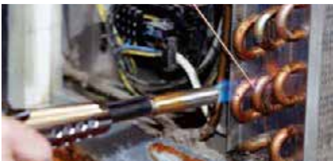
Brazing in refrigeration / air-conditioning technology
