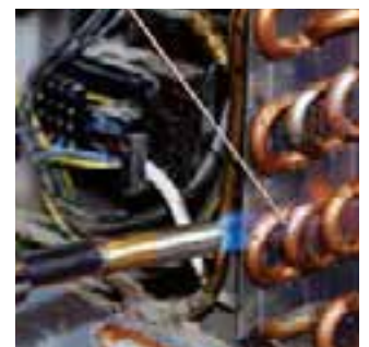
Brazing in refrigeration / air-conditioning technology
