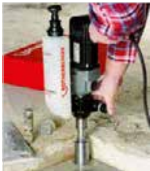
Drilling of the hardest materials
