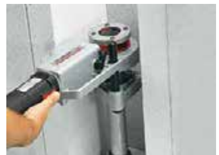
Work in confined spaces
