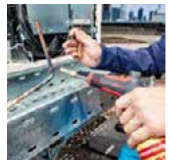
Brazing in refrigeration / air-conditioning technology
