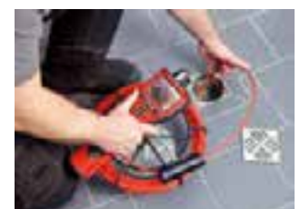
Inspection of floor drains
