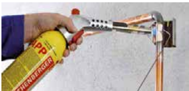
Brazing in gas installation
