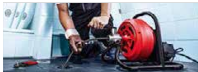
Cleaning of floor drain with 13 mm spiral
